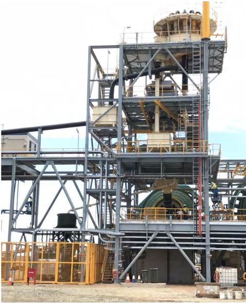
The Dacian Mount Morgans Project in Western Australia is a traditional gold plant utilising the proven option of crushing – milling – gravity circuit – CIL circuit, together with the proven option of utilising an experienced Australian engineer and contractor: GR Engineering Services.
